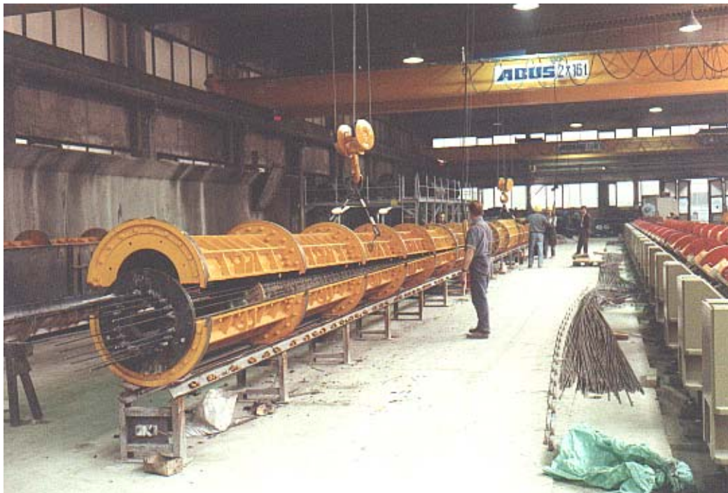
Fig. 7 Mounting the upper half of the steel mould
