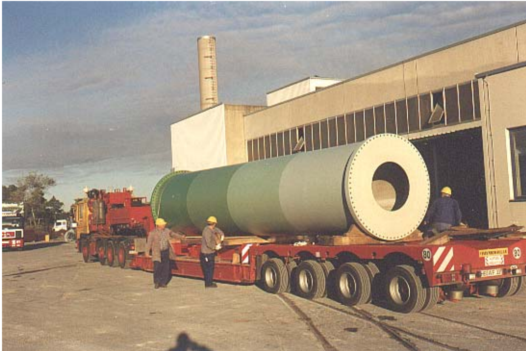
Fig. 10 Lower section of a spun concrete wind-energy tower
